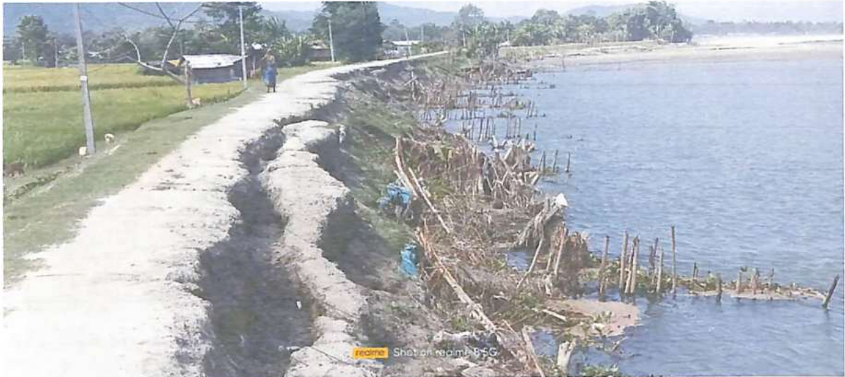
BEFORE EXECUTION EMBANKMENT
