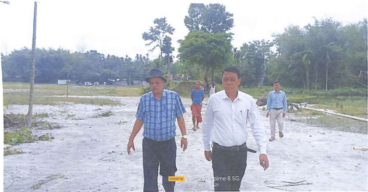
BEFORE EXECUTION AT BREACH LOCATION
